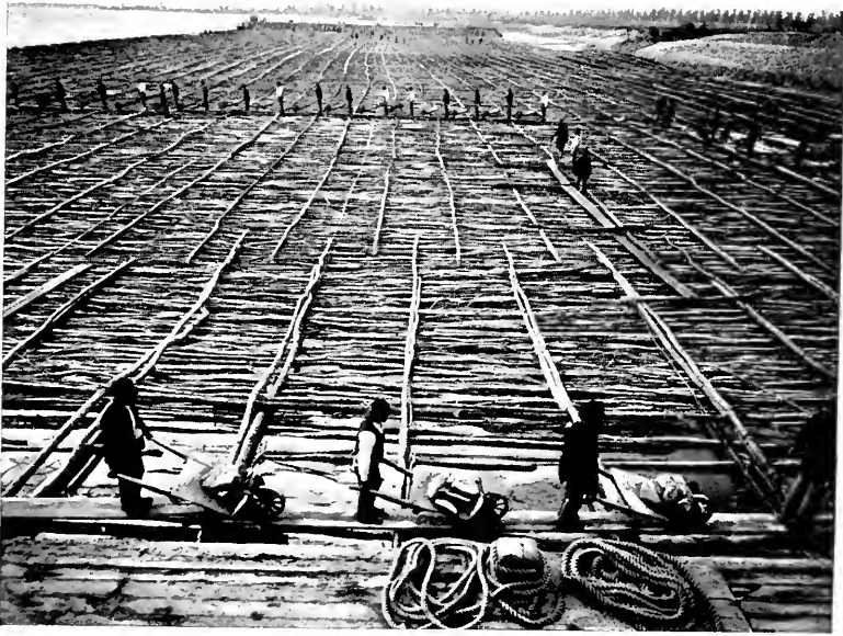
FASCINE MAT COMPLETED, READY FOR SINKING.
